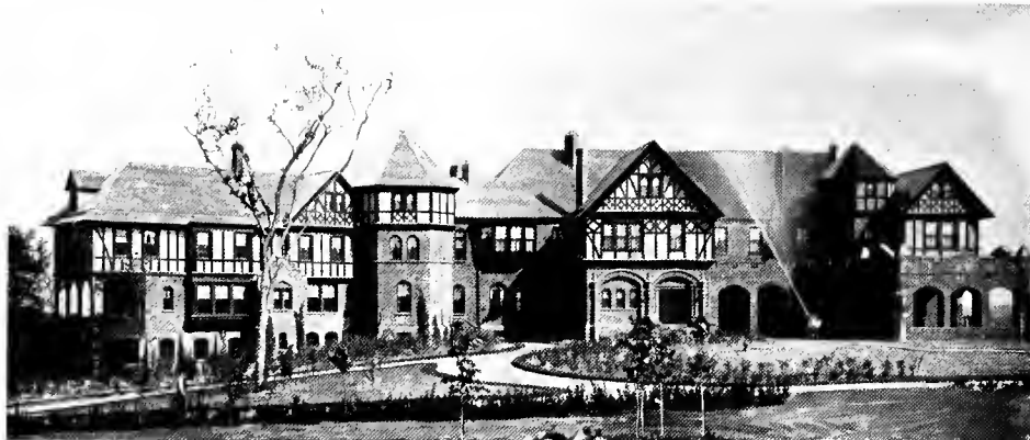
Residence of Mr. Anton G. Hodenpfl, Locust Valley, L. I., in which a Deming Water System of large capacity is installed
